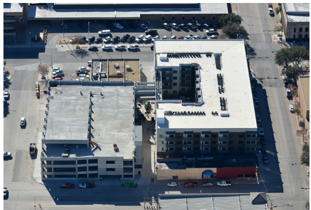
Wall Street Lofts & Public Parking Project
