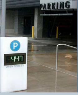
Clear signage and real-time availability for entry to parking garages. Typically, public parking spaces within a private parking garage are a percentage on the lowest levels. A centralized system and a smartphone app are likely to integrate the counting system with the driver, as well as for processing payments.
